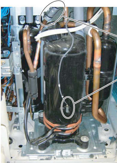
Discharge temp. thermistor (TH1)
