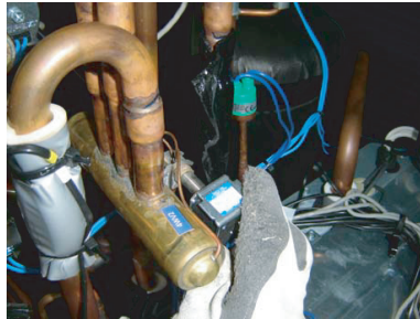
Remove the SOLENOID COIL.
