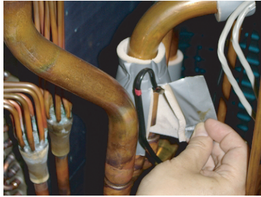
Remove the heat insulation.
