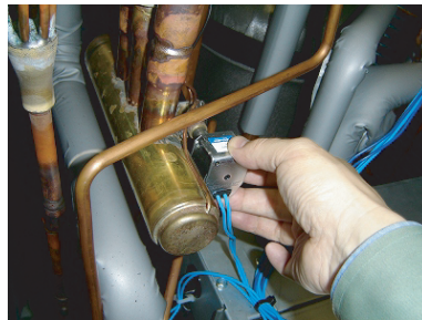
Remove the SOLENOID COIL.
