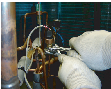
Remove the PRESSURE SENSOR with wrench.
