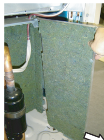
Remove the COMP BOX R by sliding toward.
